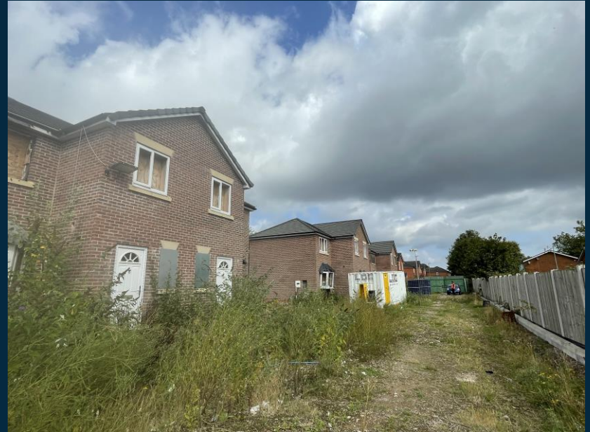
Residential development site, Sorrel Way, Clock Face, St Helens, WA9 4YN
